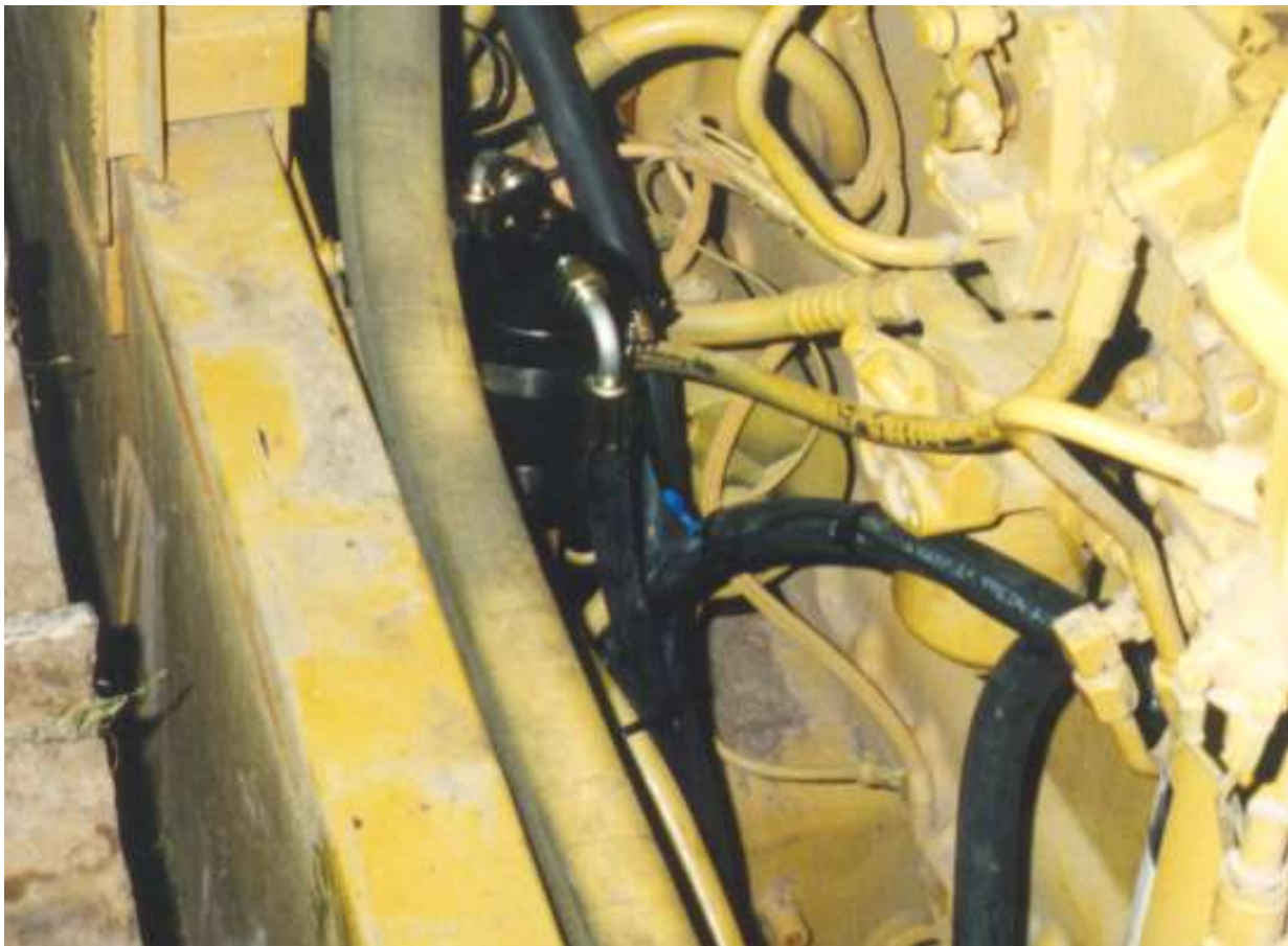
Drier in location with hoses run.
